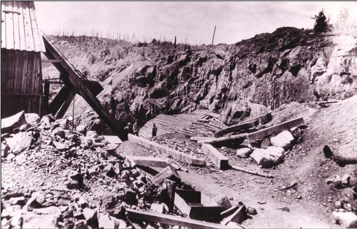
**Figure 2-2 Shaft Construction at Creighton Mine**
